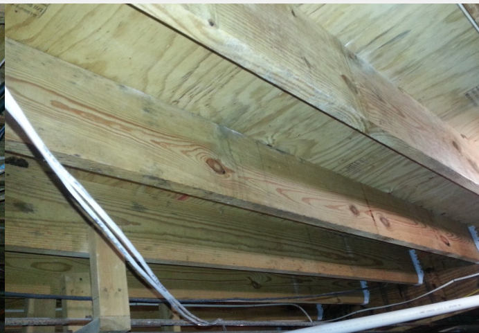
After: Treated and protected with UltraBan-PRO
